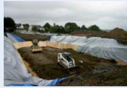
Stage 5: Fill the cell with the knotweed infested soil. No other material, contaminants, or wastes should be included.
